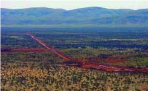
This image, which was taken in August 2001, shows the workshop area and one of the borrow pits used for the rail construction.
